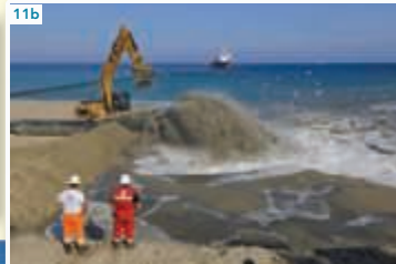
11b Dredgers pump sand through a hose to replenish beaches on Spain's Mediterranean coast, a popular tourist destination. Near Barcelona, pictured here, sand is frequently eroded during storms; natural replenishment is limited by structures that block longshore currents.
