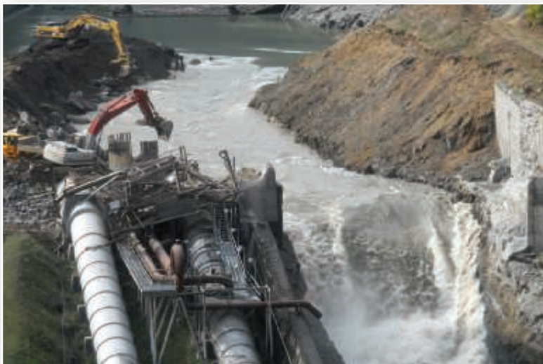
(c) Dam removal on the Elwha River, Washington
