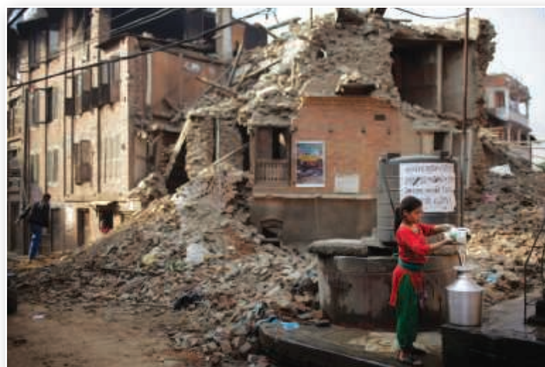
(b) Destruction in Nepal from a 2015 earthquake.
